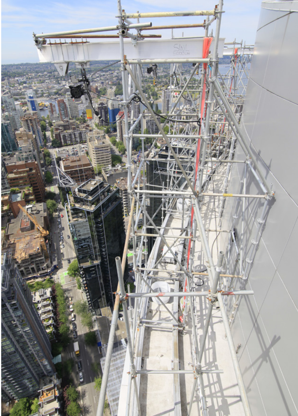
The custom platform is a 4'x400' long, multi-point suspended work platform that weighs 18,368 lbs.
